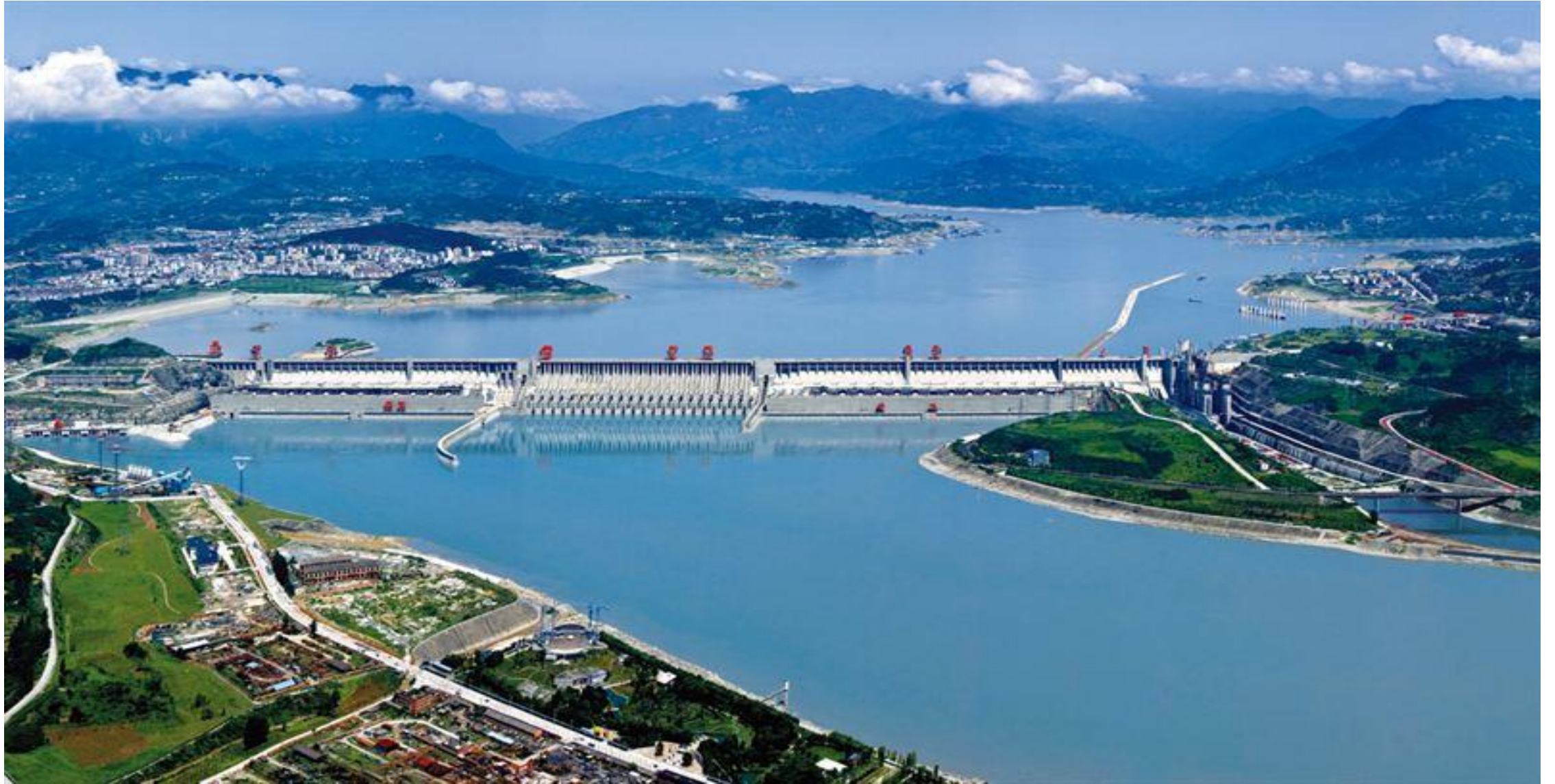
Hydro Electric Power Plant
